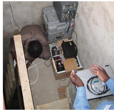
AfricaArray seismic stations in Dodoma, Tanzania (top left) and Zomba, Malawi (top right and bottom). Top right photo was taken looking down into the 3-m deep seismic vault shown in photo at left at the Geological Survey in Zomba, Malawi. Top left photo was taken looking down into the 4-m deep vault at the Geological Survey in Dodoma, Tanzania. Photos credit: Andy Nyblade.
