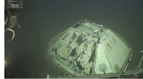
Site M09B showing evidence of having been hit by a trawler.
