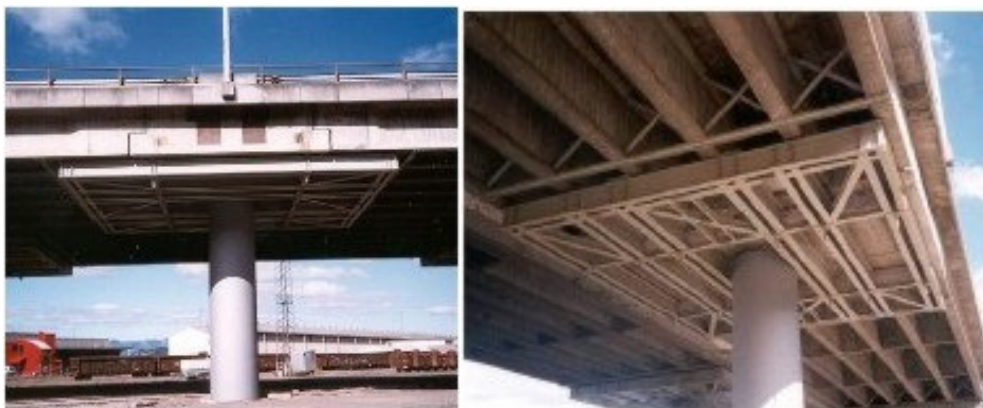
Figure 2.3. Column piers either side of where the Wellington Fault cuts the line of the Thorndon Overbridge have retrofitted “catch frames” with the capacity to accommodate lateral fault displacement of the order of 4-5 m between piers and prevent span collapse in the event of surface rupture of the fault. Photos: Billings, I.J. and Powell, A.J. (1996).
