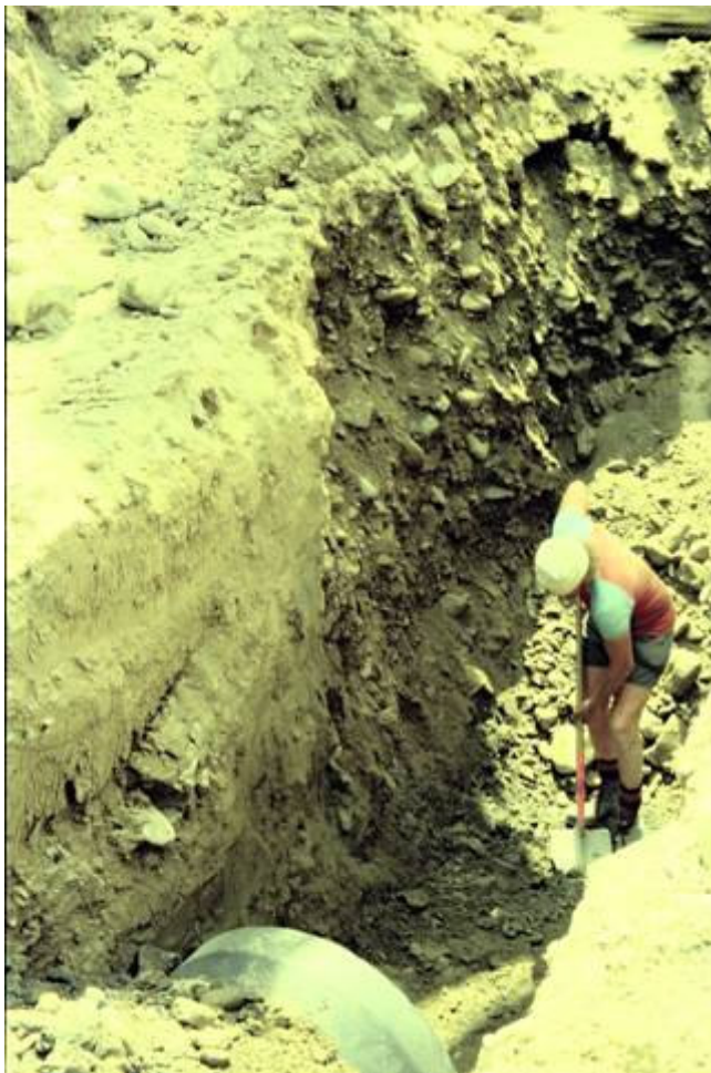
Figure 7.6. Top photo , Storm-water pipeline excavation across the Wellington Fault scarp at Harcourt Park (view looking west-southwest). Bottom photo , exposure of Wellington Fault in pipeline excavation. Fault has a sub-vertical dip and separates coarse alluvial gravel in the background (NW) from massive silt in the foreground (SE) (view looking west-northwest). Photos: Ken Thorpe.
