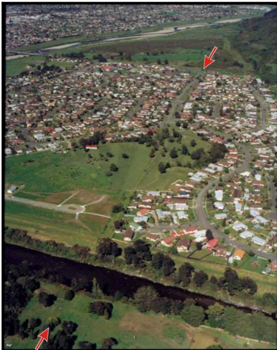
Figure 7.1. The location of the Wellington Fault (between arrows) at Totara Park was known before development of the subdivision. Note the dual carriageway of California Drive with houses on each side set back from the fault. California Park, a recreational reserve (see also Figs. 7.2 & 7.3), is also used to mitigate rapture hazard. In the foreground on the northern side of the river, preservation of the Wellington Fault scarp was one of the wishes of the person who donated Harcourt Park to Upper Hutt City Council.
