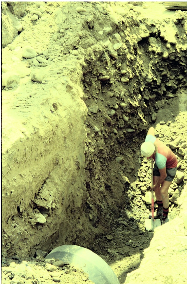
Figure 3.6. Top photo , Storm-water pipeline excavation across the Wellington Fault scarp at Harcourt Park (view looking west-southwest). Bottom photo , exposure of Wellington Fault in pipeline excavation. Fault has a sub-vertical dip and separates coarse alluvial gravel in the background (NW) from massive silt in the foreground (SE) (view looking west-northwest). Photos: Ken Thorpe.
