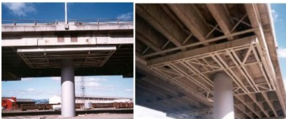
Figure 1.3. Column piers either side of where the Wellington Fault cuts the line of the Thorndon Overbridge have retrofitted “catch frames” with the capacity to accommodate lateral fault displacement of the order of 4-5 m between piers and prevent span collapse in the event of surface rupture of the fault. Photos: Billings & Powell (1996).
